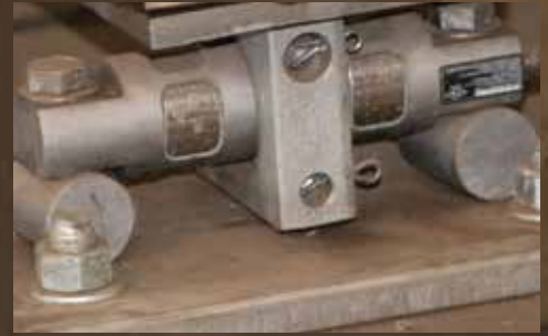
FM-approved load cells are installed under the distillery’s 6,000+ gallon, stainless steel storage tanks.
